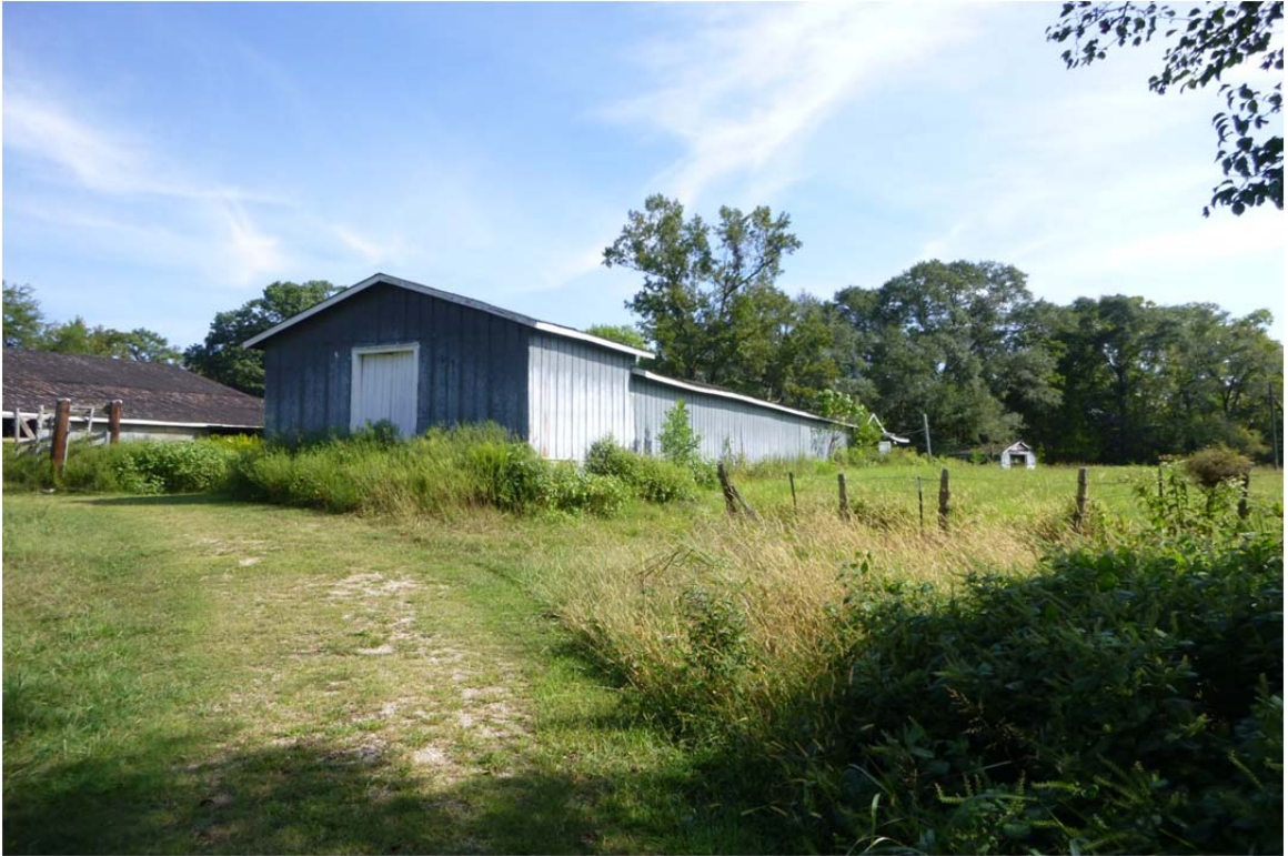
Figure 3. HAR 1, cross gable barn. View northeast.
