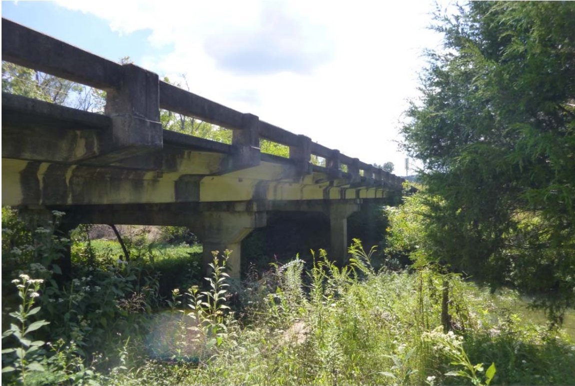
Figure 9. HAR 2, BIN 3128. View southwest.
