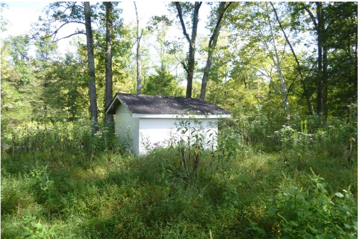
Figure 8. HAR 1, wellhouse. View northeast.
