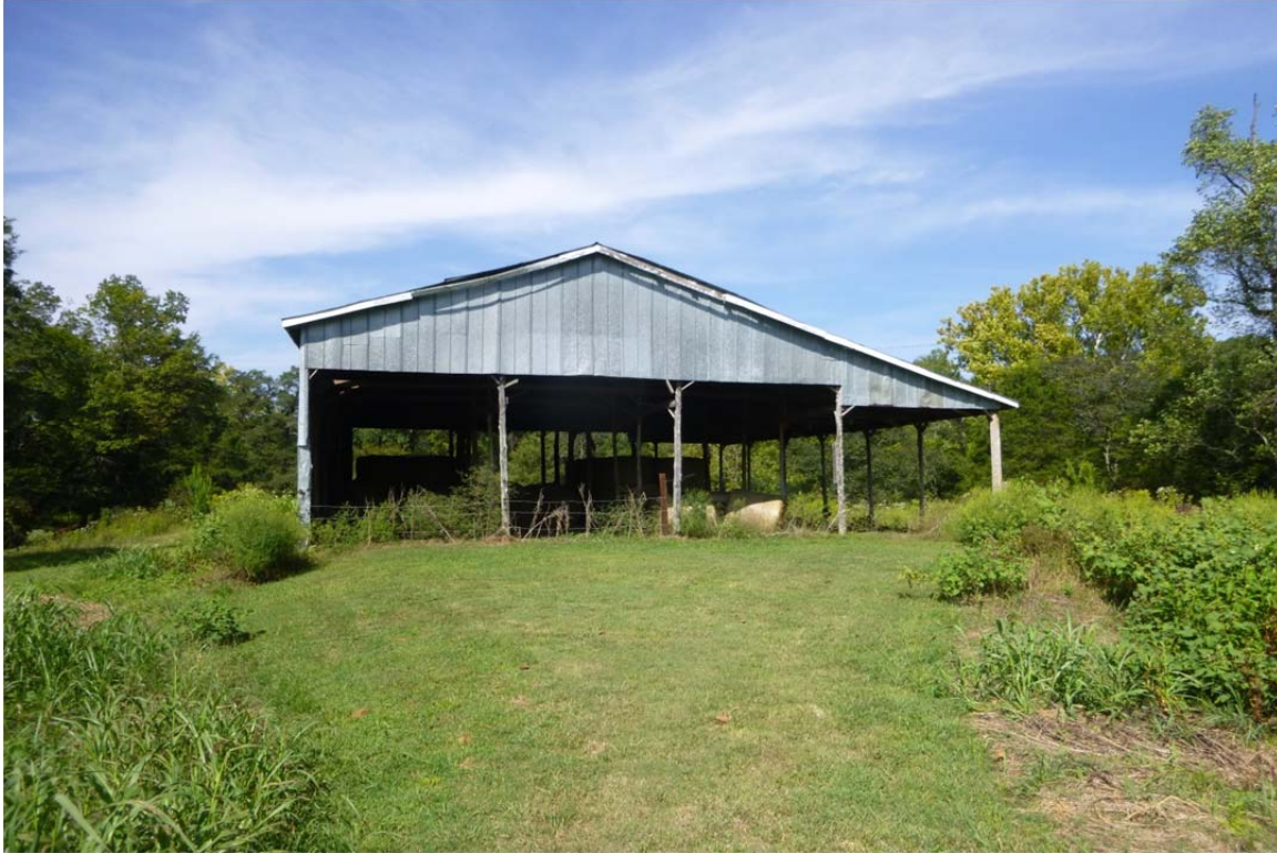
Figure 5. HAR 1, gable roof barn. View northwest.
