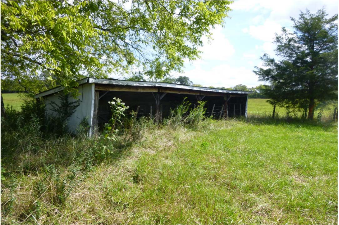
Figure 7. HAR 1, vehicle shed. View east.
