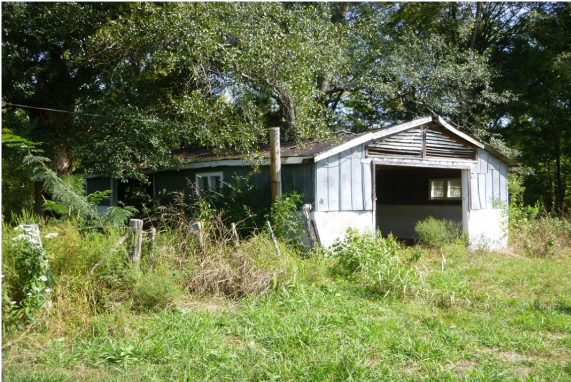
Figure 6. HAR 1, concrete block vehicle shed. View northeast.
