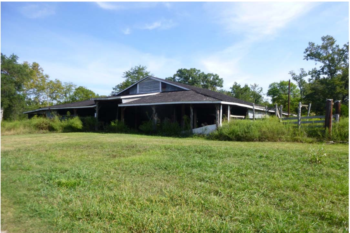
Figure 4. HAR 1, gable on hip roof barn. View northeast.
